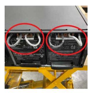
F. Install batteries into external battery pack chassis, battery handling is the same as we handle internal batteries
