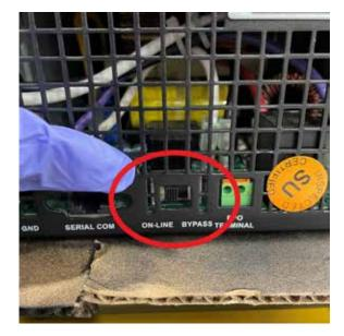
PLEASE NOTE: While in bypass there is a slight risk of the load dropping due to a power failure or an unforeseen internal failure of the UPS.
