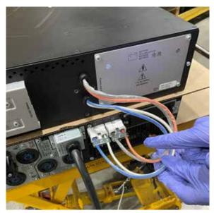
K1. All the connections are now completed. Plug UPS power cord into the wall outlet and the fan should power on. Now press the O button on the front display bezel and the Online LED will begin to blink. Once the blinking stops the UPS is now operating properly.
